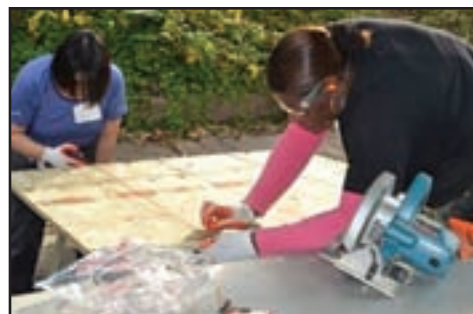
Volunteers assist with the playground reconstruction on Oakwood Avenue
