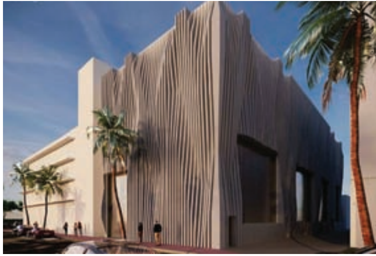
A new Alton Road substation would be open by the end of 2021.
