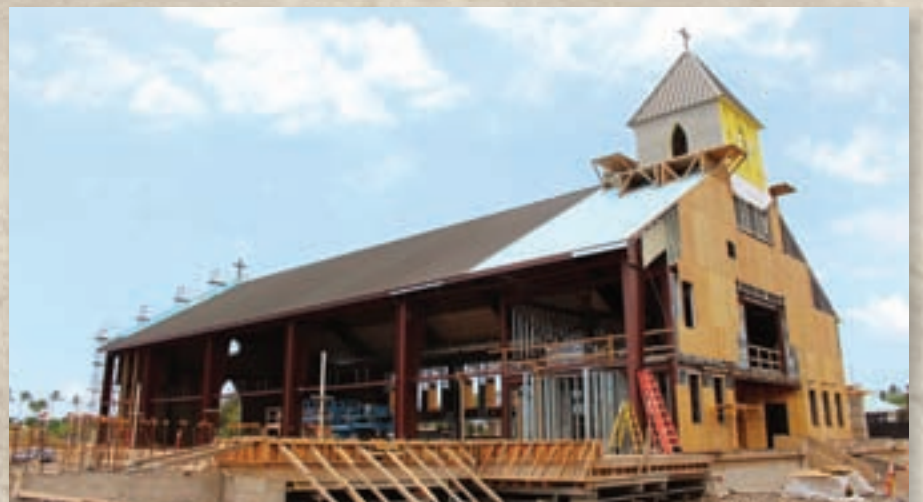
St. Michael the Archangel Church, Kailua-Kona – under construction
