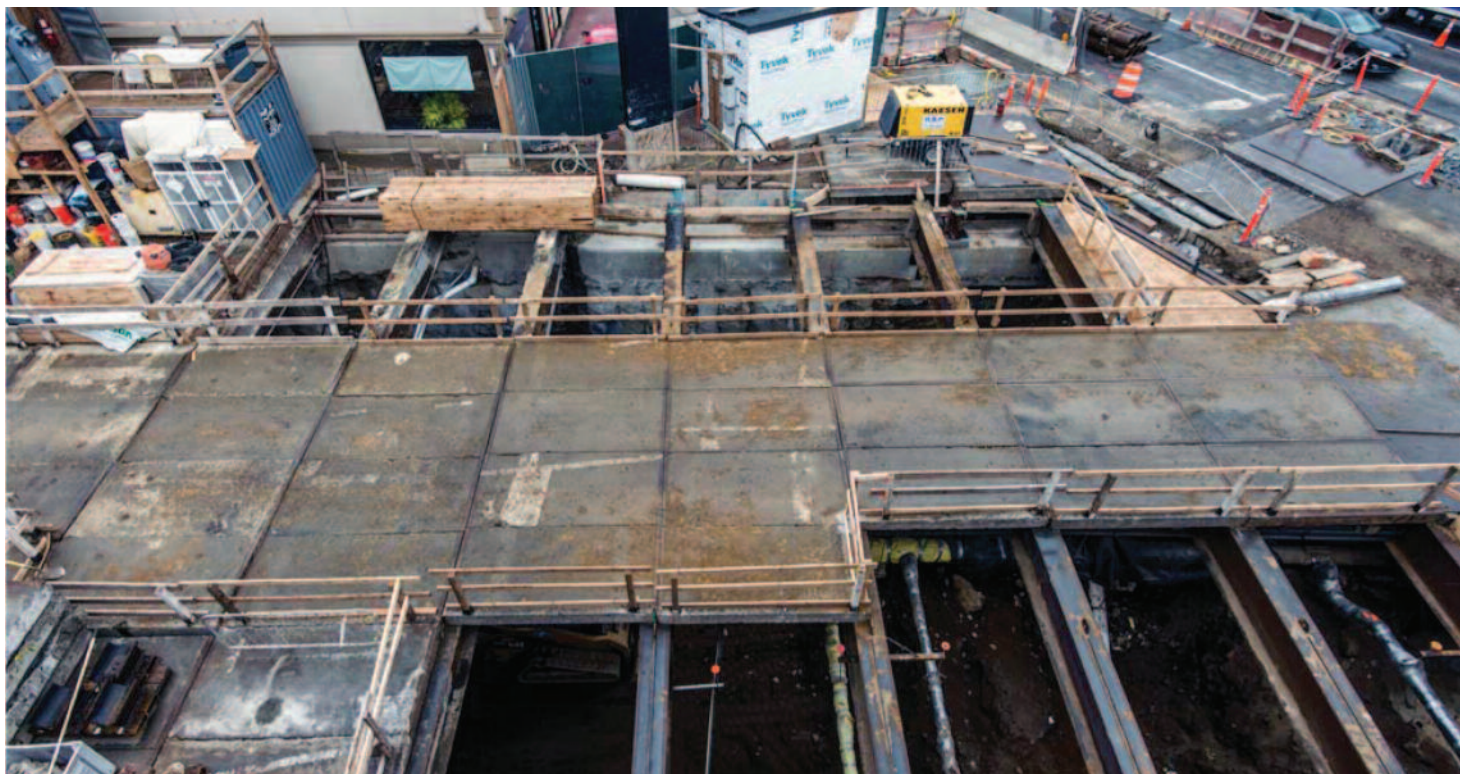
Posillico installed a modular road decking system supported by a secant pile wall support of excavation. This allowed for low headroom excavation and bracing while maintaining traffic and access for emergency vehicles.
