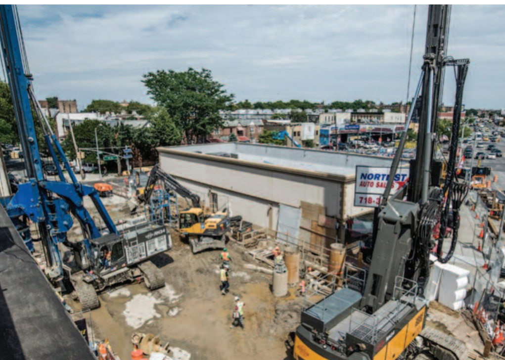
In The Dry – Installing the lower level of bracing. Moisture on the secant pile wall give an indication as to the height of the groundwater table.
