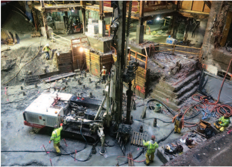
Photo 14: Casagrande C-8 drilling core piles.
