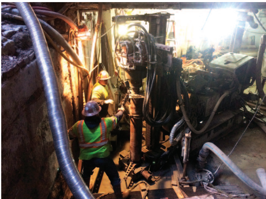
Photo 11: Drilling in tight places with minimal access.
