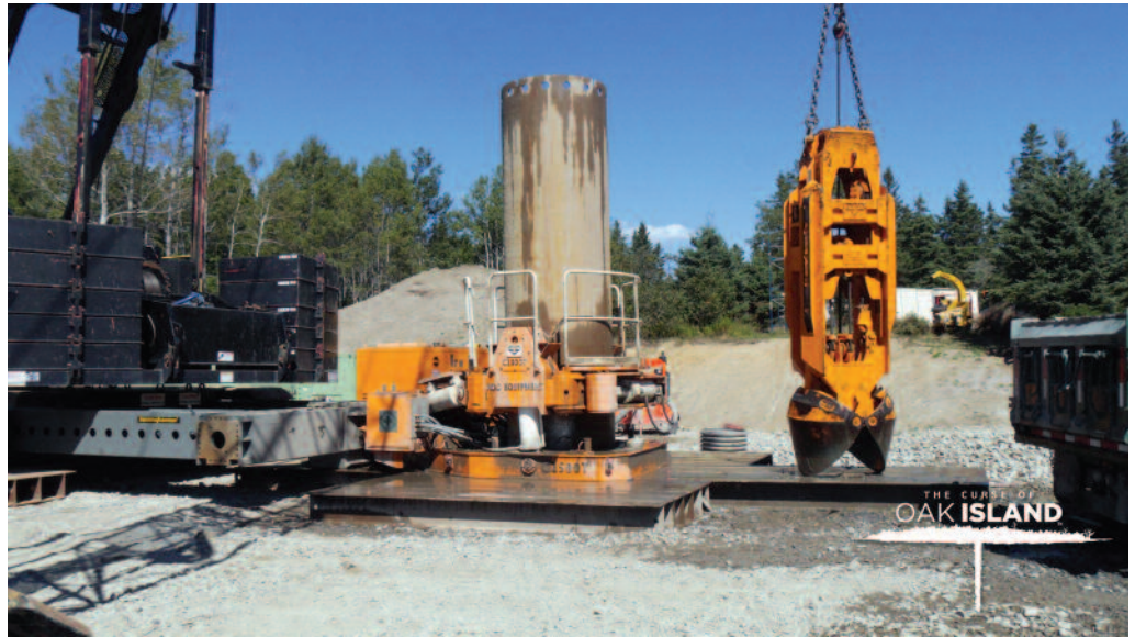
Shafts were excavated by means of a BUMA hammer grab. The oscillator was attached to the crane by a custom bridge by Bermingham.
