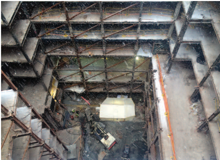
Photo 10: Casagrande C-8 drilling core piles within the central core while a snow storm hammered Boston outside.
