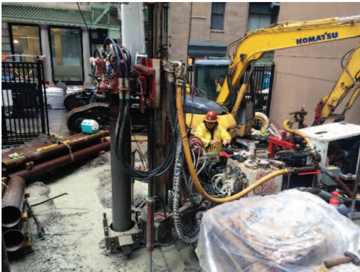
Photo 4: Dk-525 drilling compression test pile.
