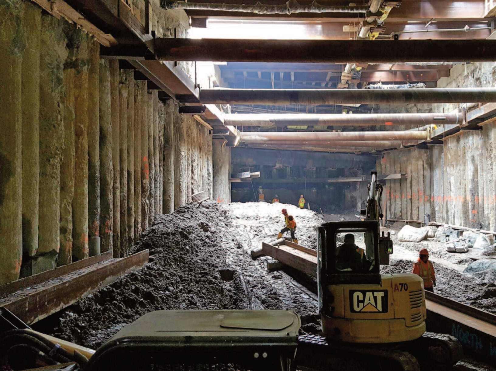
In The Dry – Installing the lower level of bracing. Moisture on the secant pile wall give an indication as to the height of the groundwater table.
