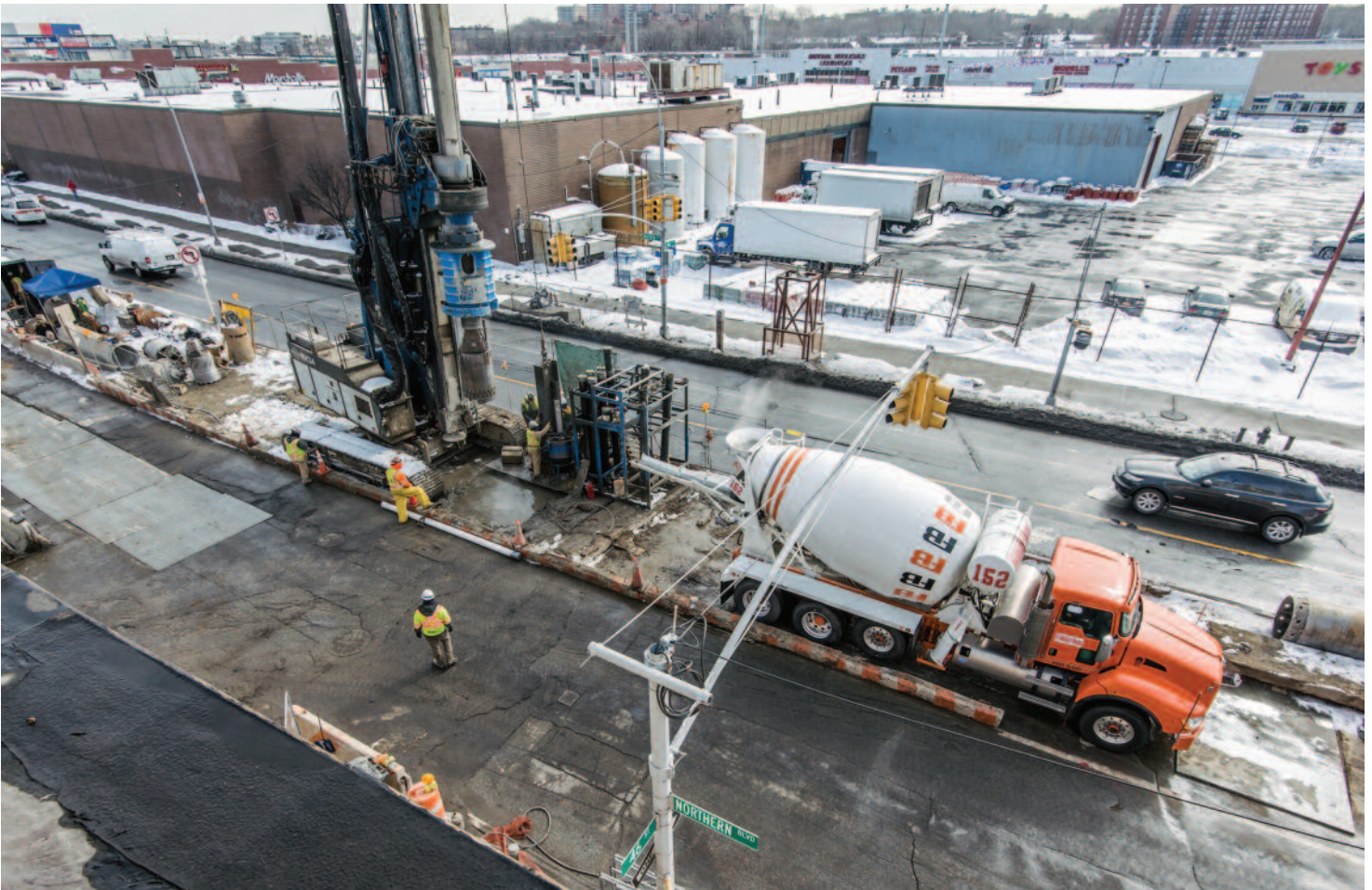
Inching Across Northern Boulevard – The underground structure crossed Northern Boulevard – a main commuting thoroughfare – so the work from up top had to be performed in narrow work zones while traffic passed on either side.
