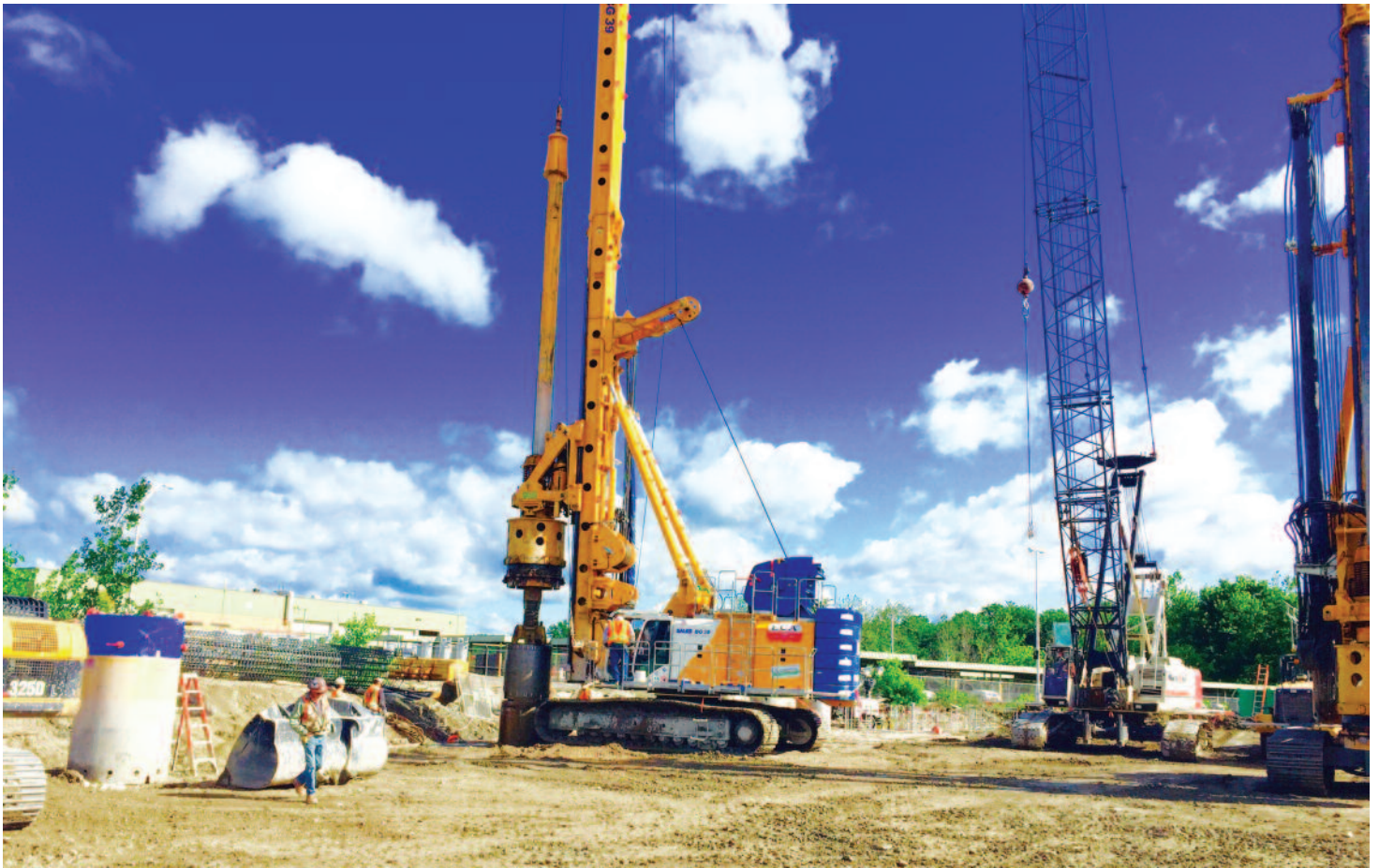
Bauer BG 39 Drill with 38-Ton Single Layer Winch.
