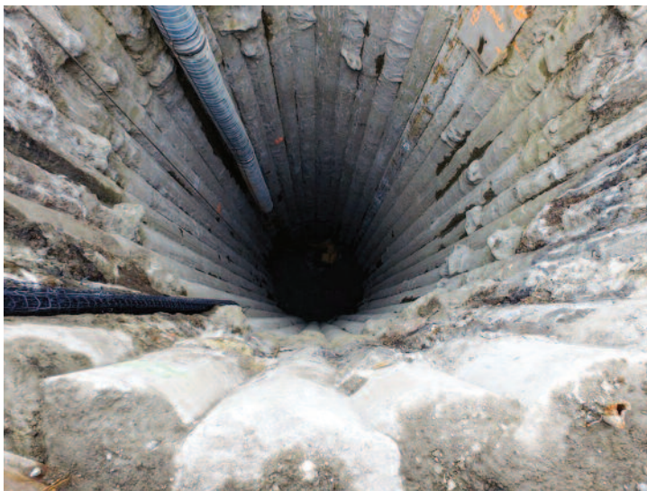
Secant pile wall at Dugway Storage Tunnel in Cleveland.
