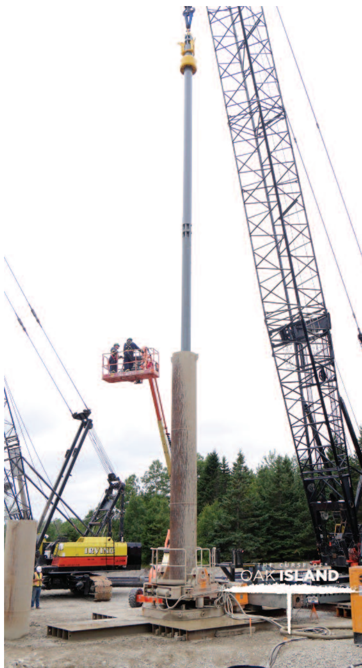
Birmingham's flying lead used in conjunction with ROC's C1500T oscillator.
