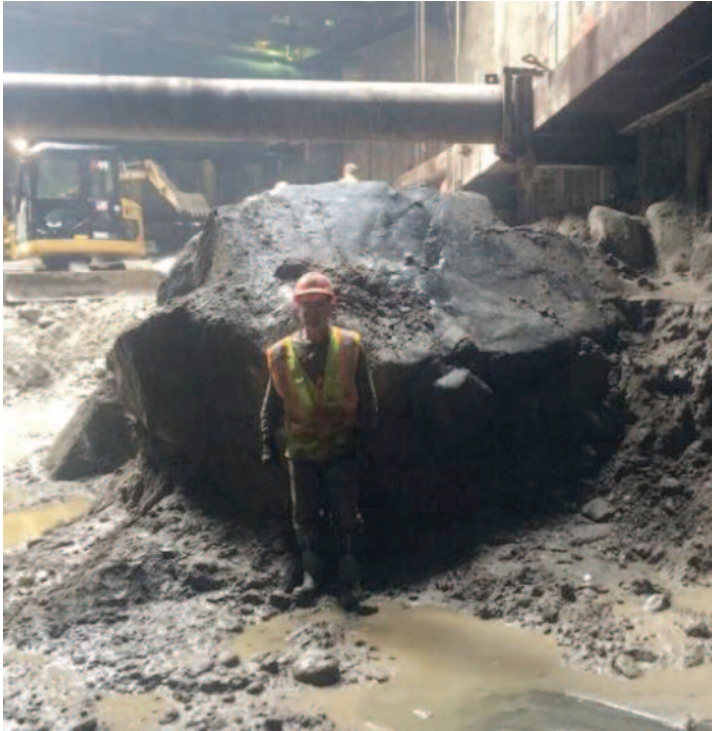
Big Boulder – “Drilling in this part of Queens can be challenging, with multiple boulders per hole and some as much as 13 feet thick, this site lived up to the area’s reputation,” says James Myers, P.E., Project Manager for Moretrench.
