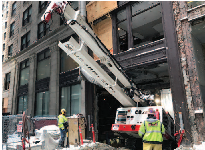
Photo 2: The Casagrande C-8 entering the building off Quaker Lane. A hole was created in the outer wall just big enough for the C-8 to enter. The length of the mast had to be factored into the required clearance when walking down the ramp to 25 feet (7.3 meters) below street level.
