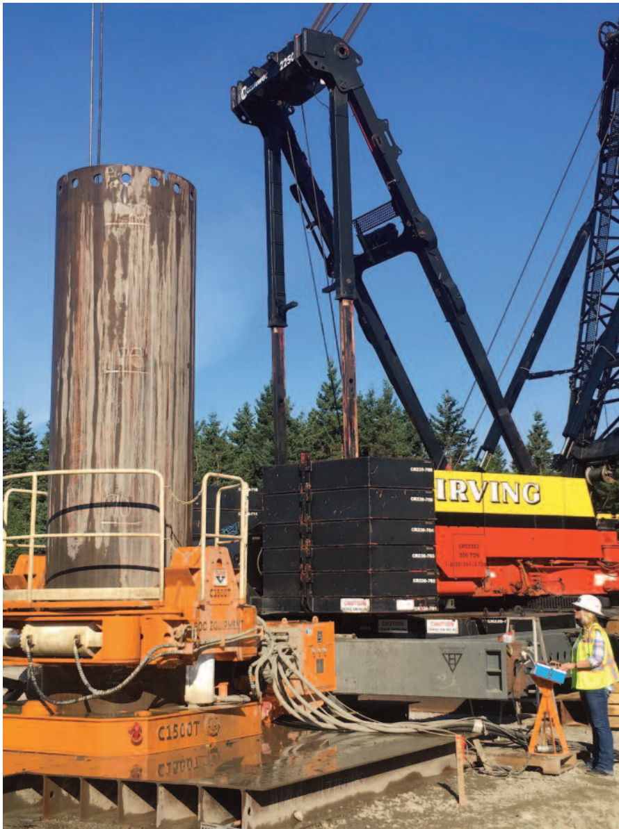
ROC Equipment's Vanessa Lucido operating ROC's C1500T oscillator.
