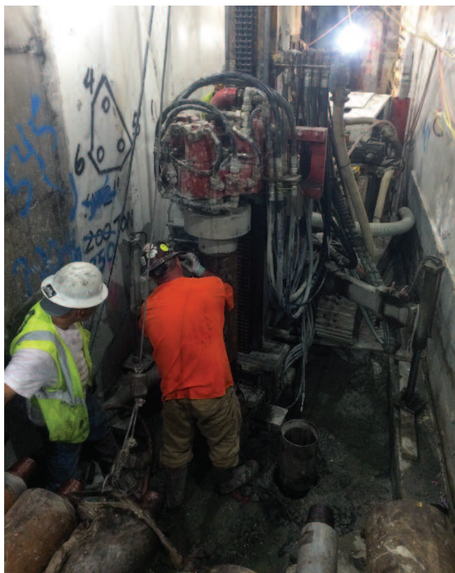
Photo 12: Drilling in a narrow corridor.
