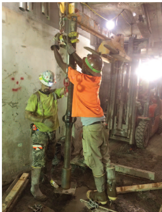
Photo 13: Installing pile reinforcing with a fork truck while piles are drilled elsewhere.
