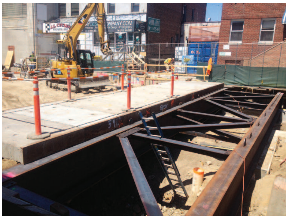
Detail of the Decking Construction – Most of the excavation and all structural concrete work and mechanical installations were performed below a panelized decking system supported by the secant pile wall.
