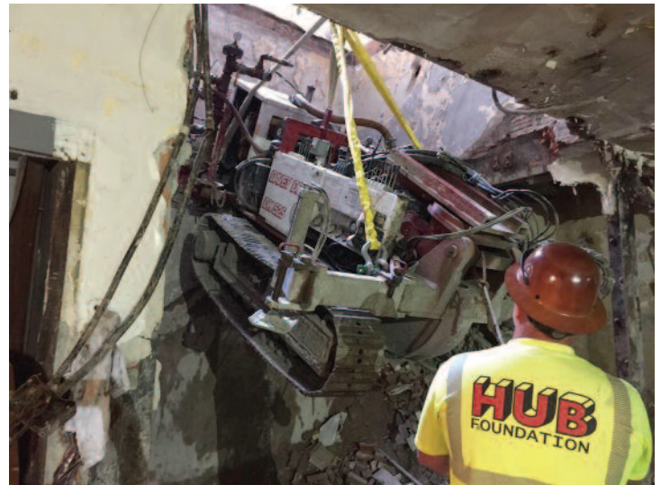
Photo 1: The DK-525 low headroom drill rig hoisted into the building through a small hole in the street.
