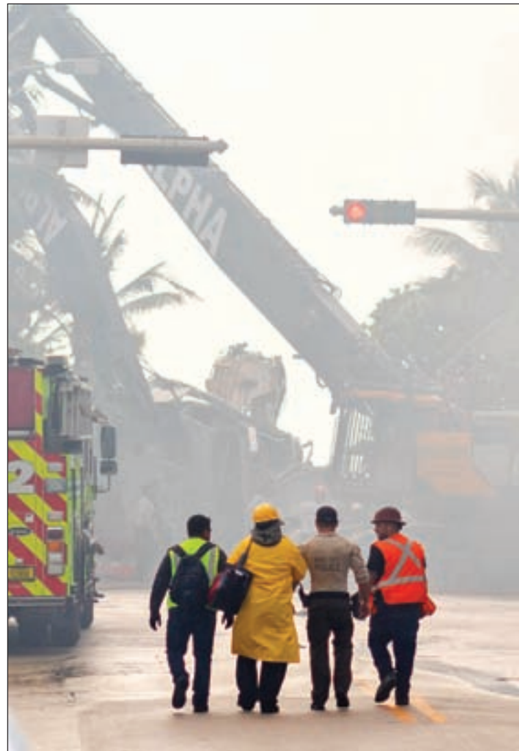
Fire rescue and search specialists walk toward the partially collapsed Champlain Towers South in Surfside June 25, 2021, the day after the tragic event in Miami Beach. (TOM TRACY | FC)
